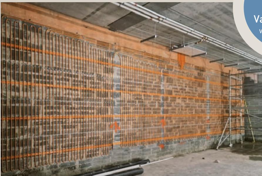
The EasyFlex wall heating/cooling is highly energy-efficient and easy to install.
