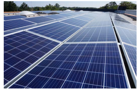
Electricity will be generated on the premises to power the production machines as well as office and storage rooms.
