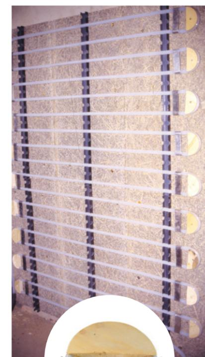
The first bending model for the first system walls was affixed to the pipe on the wall and plastered over
